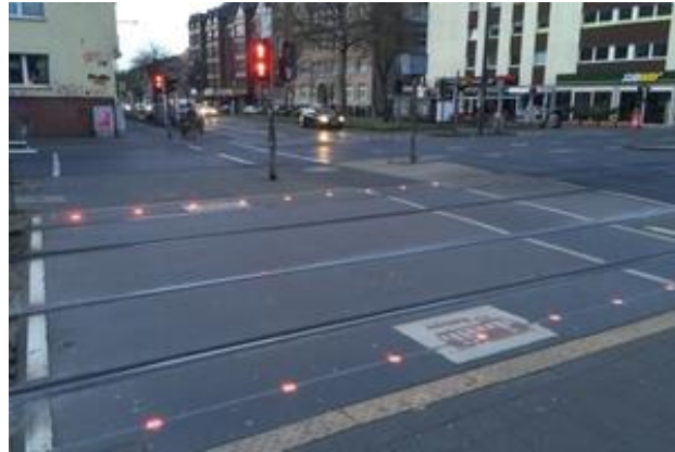
Fig. 4. Ground warning lights
