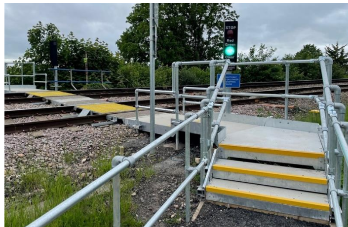
Fig. 5. Pedestrian crossing over the railway track [17]
